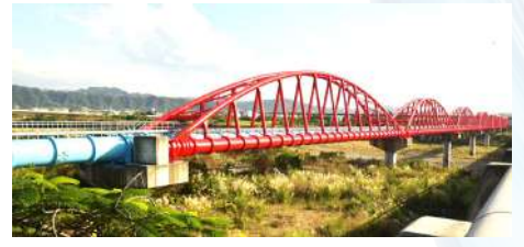
后豐大橋水管橋工程完工 Completion of Hofong Bridge Aqueduct Project
