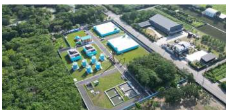
屏東內麟淨水場新建工程 - 土建完工 Completion of Pingtung Nei-Lin Water Treatment Plant Project
