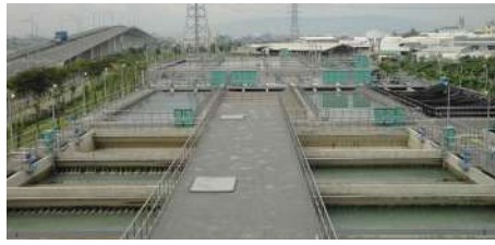
南部科學工業園區～高雄園區供水工程完工 Completion of the Water Supply Project for the Southern Taiwan Science Park- Kaohsiung Science Park
