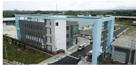
曾文淨水場擴建第一期工程完工 Completion of the Tsengwen Water Treatment Plant Expansion Phase I Project
