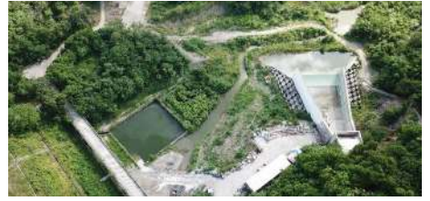
南化水庫防淤隧道工程計畫完工 Completion of the Nanhua Reservoir Desilting Tunnel Project
