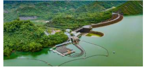
南化淨水場壩頂取水工程完工 Completion of Crest Water Intake Project at Nanhua Reservoir
