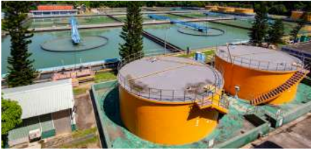
坪頂淨水場改善工程完工 Completion of Pingding Water Treatment Plant Improvement Project
