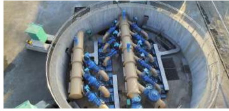
高屏溪溪埔伏流水工程完工 Completion of the Gaoping River-Xipu Subsurface Water Development Project
