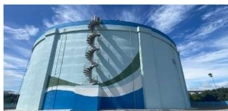
台中市聚興 4 萬立方公尺配水池工程完工 Completion of the Taichung Juxing 40,000 m 3 Water Distribution Reservoir Project
