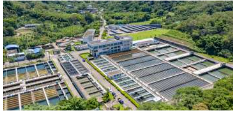
寶山淨水場第三期擴建工程完工 Completion of Phase III Expansion Project of Baoshan Water Treatment Plant
