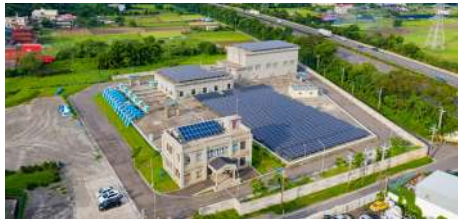
板新大漢溪水源南調桃園計畫－ 頂山腳加壓站土建工程（續）完工 Completion of Dingshanjiao Booster Pumping Station Project
