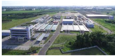
湖山淨水場新進工程完工 Completion of the Hushan Water Treatment Plant Project
