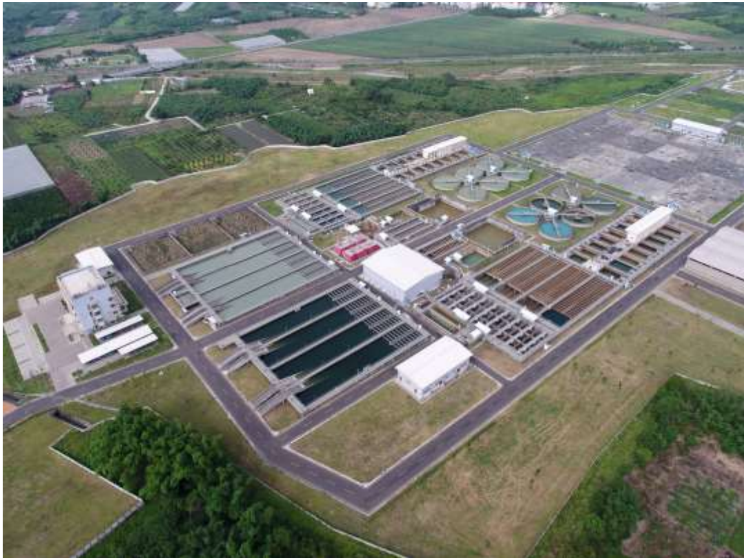
Hushan Water Purification Plant
