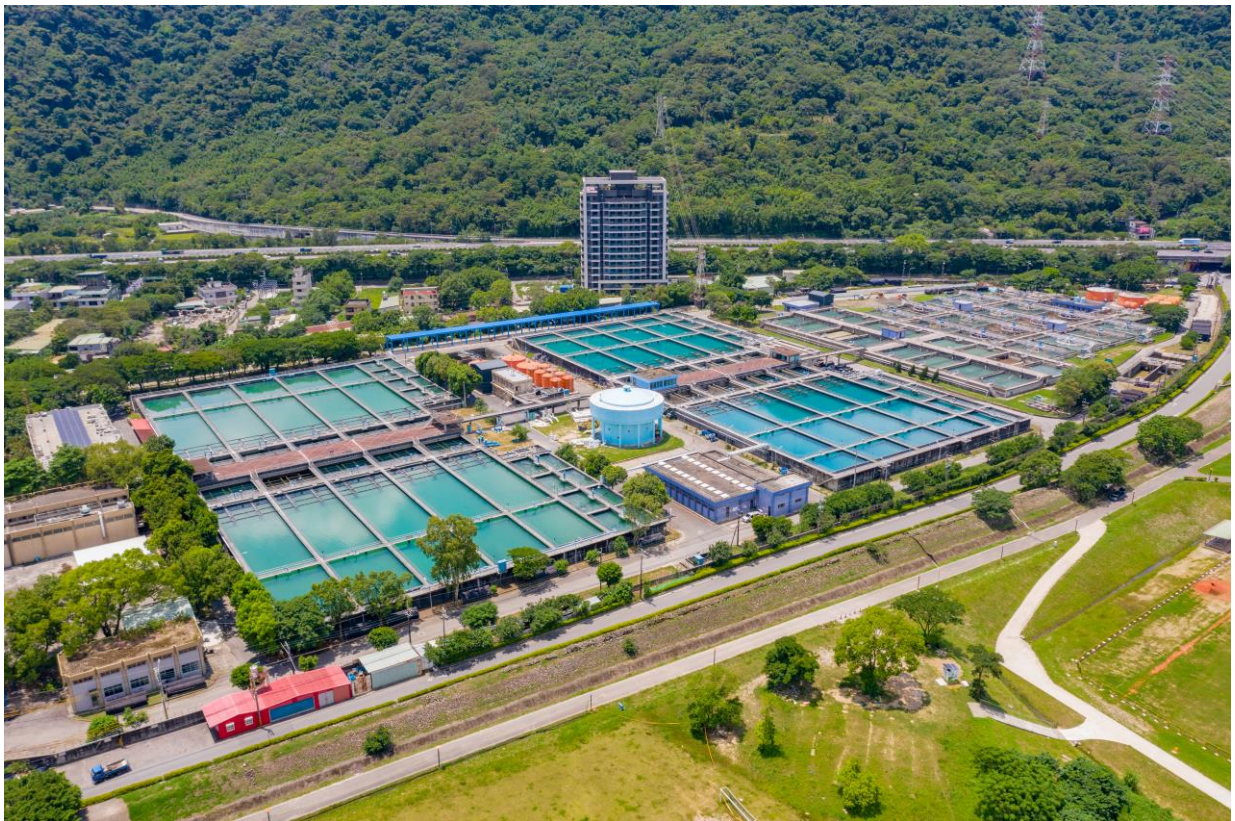
BanSin Water Purification Station
