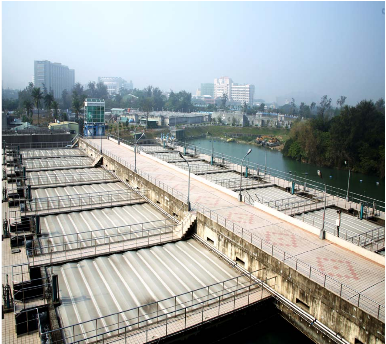
Chengcing Lake Advanced water treatment plan
