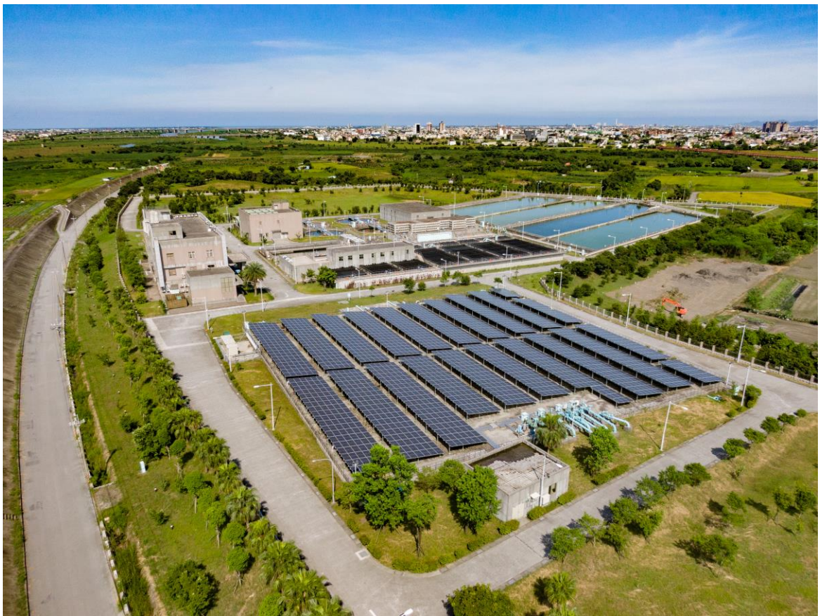
Guansing Water Treatment Plant
