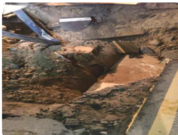
開挖確認管線漏水點
