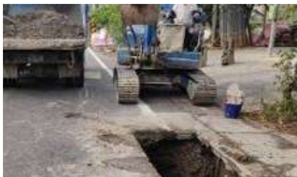
開挖確認管線漏水點
